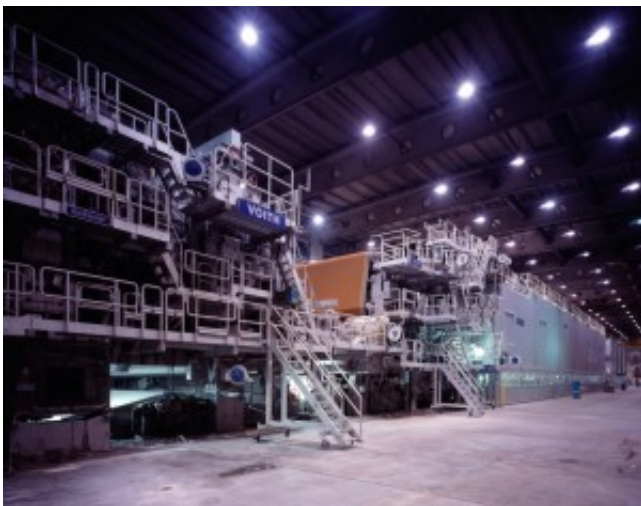
Figure 1: The paper machine is controlled via a PROFIBUS network
