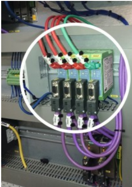
Figure 2: TH LINK PROFIBUS can be integrated without interfering with the operation of existing installations and requires very little additional space in the control cabinet.
