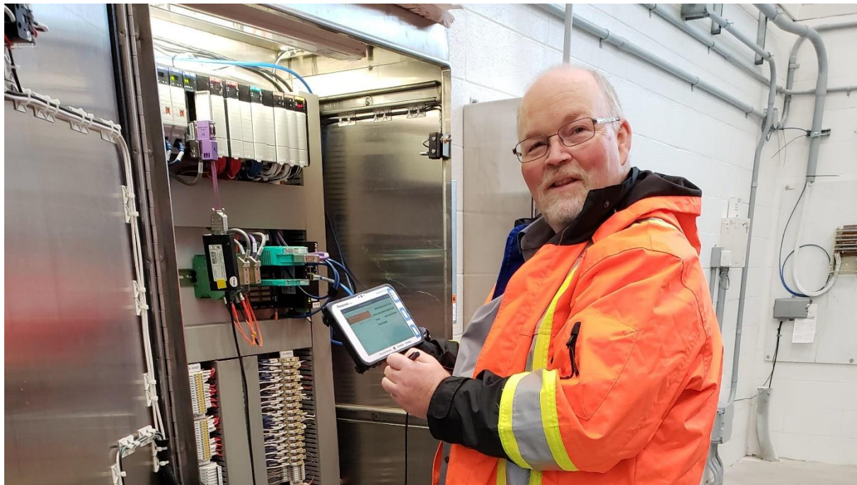
Figure 3: The author troubleshooting PROFIBUS using Osiris running on Mercury with a Proficore
